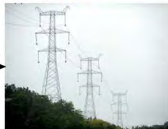
High Voltage Transmission Line
